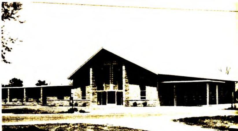
CARDINGTON, OHIO, CHURCH DEDICATED —General Superintendent Hugh C. Benner and Dr. Harvey S. Galloway , Central Ohio District superintendent, dedicated a $250,000, contemporarily designed church plant at Cardington, Ohio, June 27. The fully carpeted sanctuary will seat 350 persons. An educational unit, built around an open court or "prayer garden," is adequate for a Sunday school attendance of 500. Rev. Ellis L. Teasdale is pastor.
