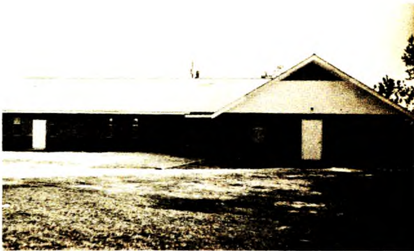
Pearl River (La.) church as it neared completion
