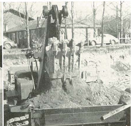
The power shovel dragging out the "hole."
