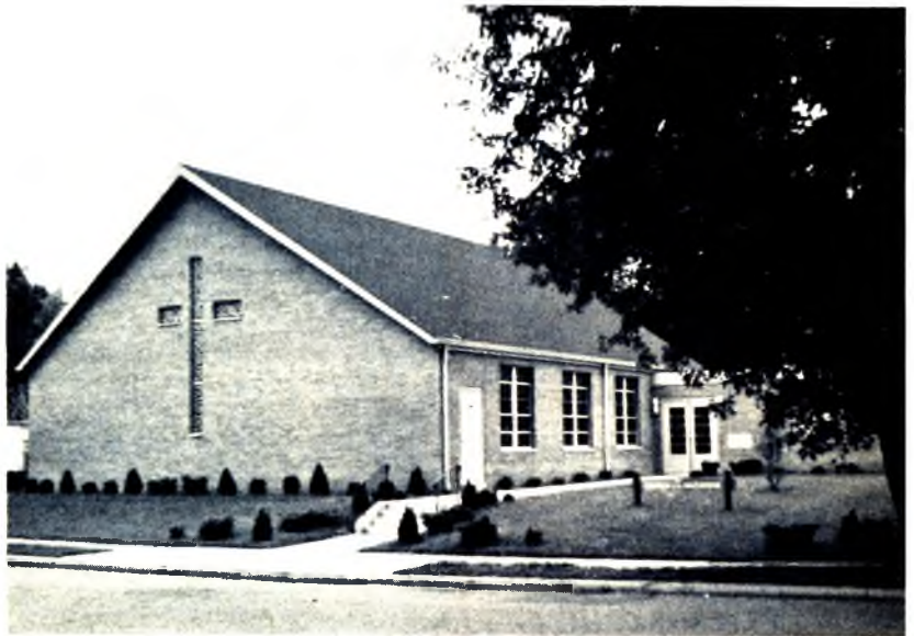
NEW OHIO CHURCH —The congregation at Chillicothe (Ohio) First Church began worshipping January 24 in its new church. The sanctuary seats 320 persons; there are 12 classrooms, plus an overflow area used for youth services, all of which are air-conditioned. Rev. Daniel McNutt is pastor.
