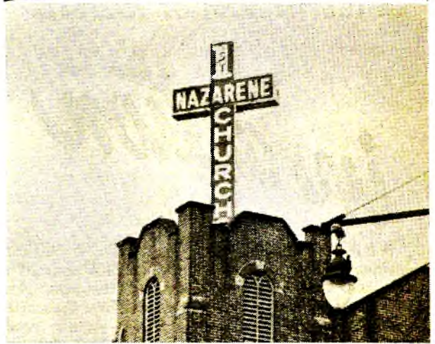
800-POUND NEON REVOLVING CROSS. The cross, sixteen feet high, is erected on top of a fifty-foot tower at the corner of Ironton's (Ohio) First Church. Sign men say this is the first revolving completely neonized cross. Rev. J. Donald Carrico is the pastor.
